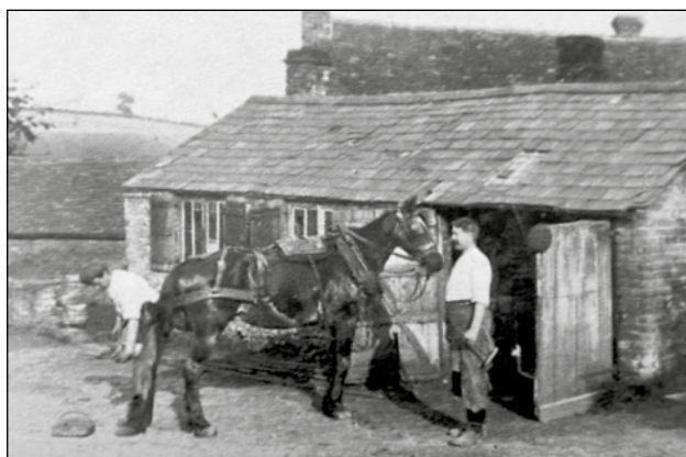
The blacksmiths at Flowers Bottom, probably around 1920. The high roof behind the smithy is the back of the Old Plough.
